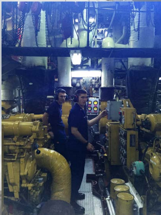
ENS Schoen commences a startup routine for the #2 Main Diesel Engine prior to it turning on.
